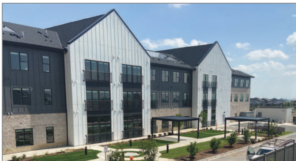
Juliet balconies safely provide direct outdoor access at The Gallery at Broomfield.
